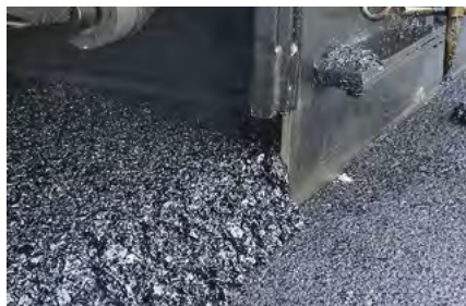
Figure 16. Laying of an asphalt mixture layer
