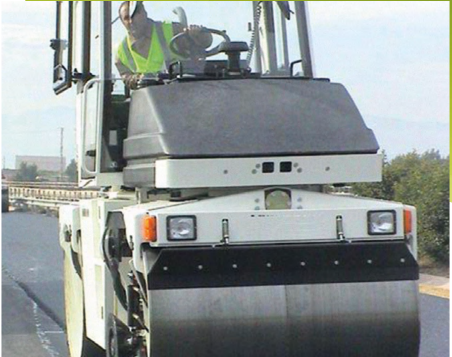
Figure 17. Compaction with a smooth roller
