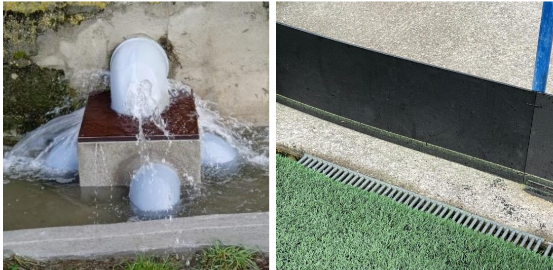
Image 11: Clogging of the filters of the general drainage manifold during short periods of heavy rain (left) and marking on the fencing panels of the water level reached during flooding (right).
