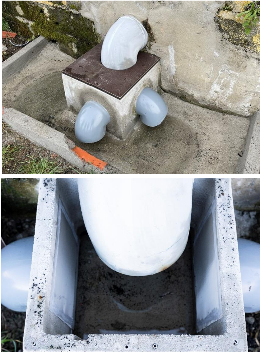
Image 4: Manhole and filters of 100 \mu\text{m} at the general drainage.
