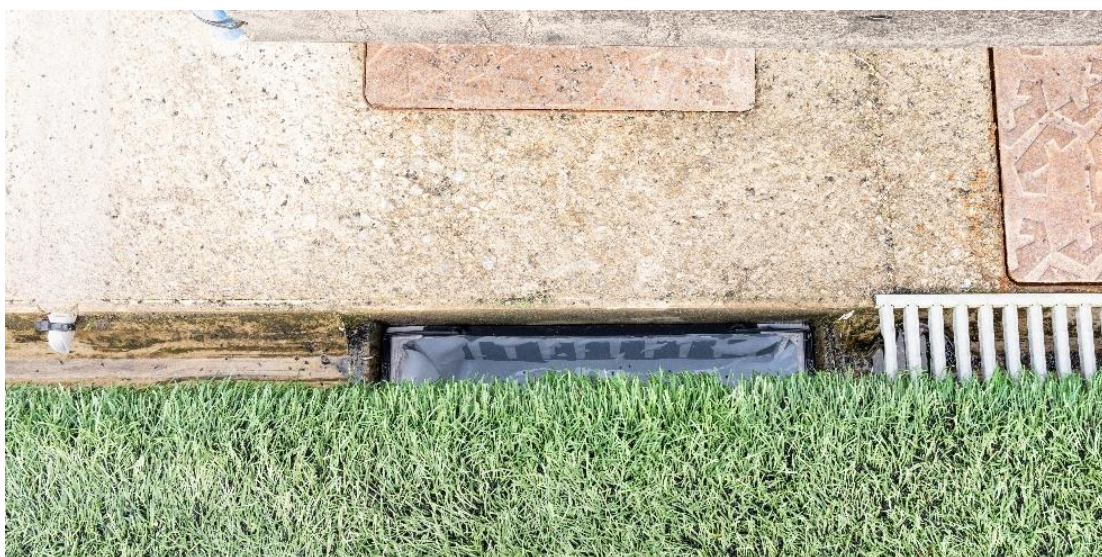
Image 3: Filters of 100 \mu\text{m} installed in the perimeter gutters.
